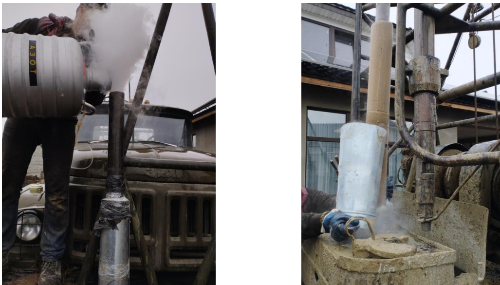
Fig. 5. Production of CGF using nitrogen with subsequent installation in the intake section of the well
